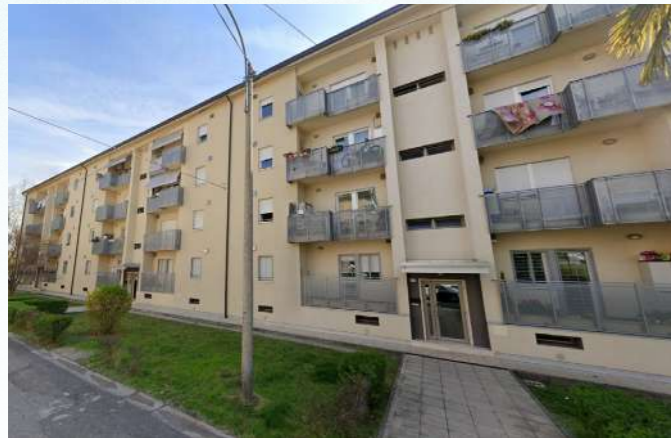
Bologna – “San Ruffillo” – Social Housing building after the refurbishment works © AESS
